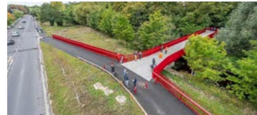
Active Travel bridge, Dodder Greenway
