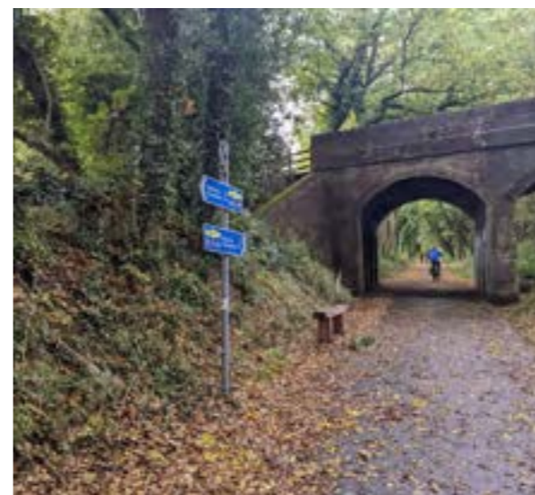
3 Cherry Tree Lane bridge
