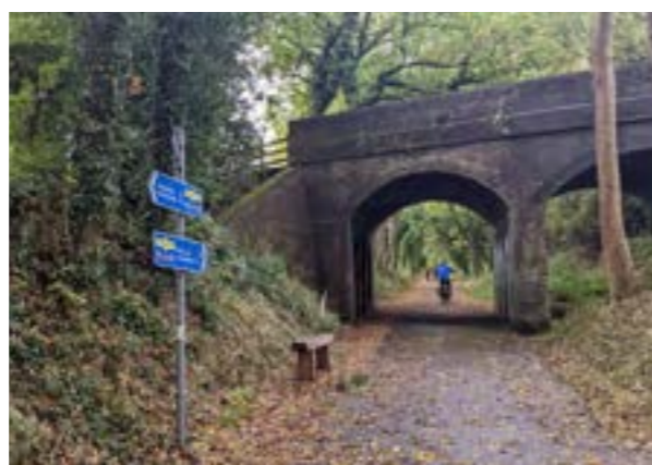
Cherry Tree Lane bridge
