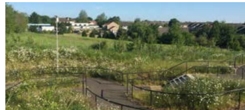
Ramp access on Loanhead Railway Path Extension, Danderhall
