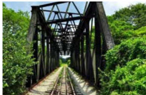
Former railway bridge
