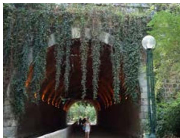
Lighting added under railway tunnels
