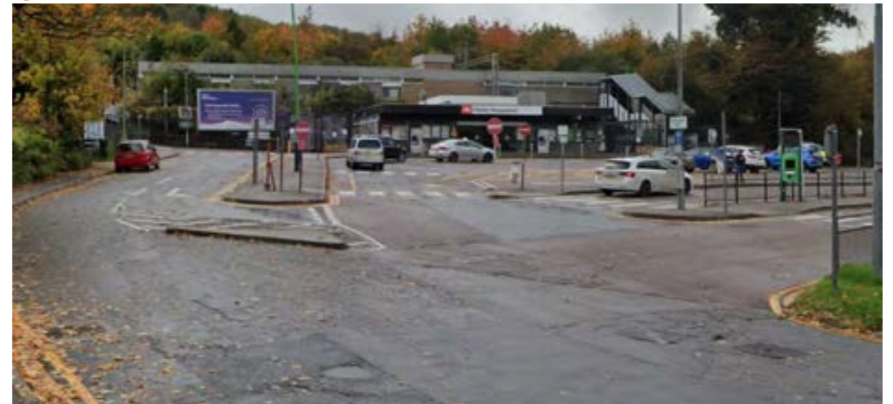
2 Narrow shared footpath on Station Rd
