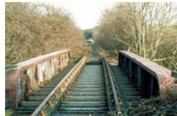
Bridge over Redbourn High Street (date unknown)
